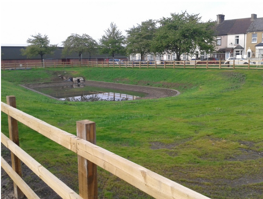
Figure 1: Drainage Pond at Gumley Road
